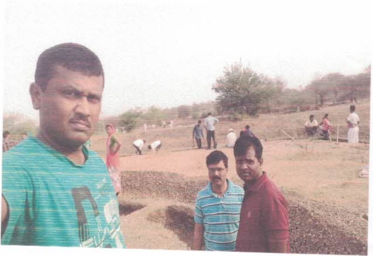
Teacher Partition in Water Foundation Work
