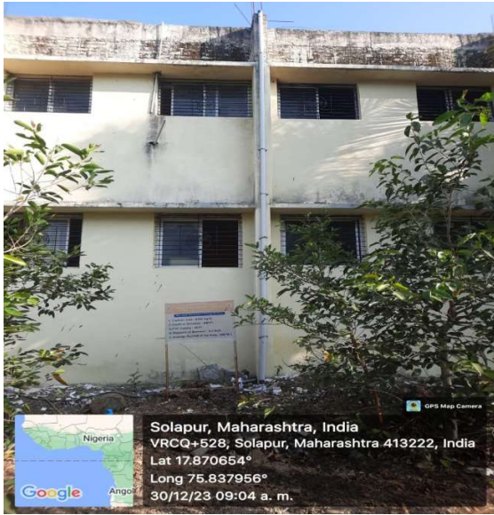
53.Rain Water Harvesting
